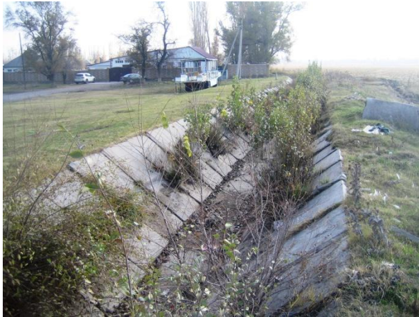
Poorly maintained on-farm canal in Chui Oblast (left) and properly maintained on-farm canal in Osh Oblast (right)
