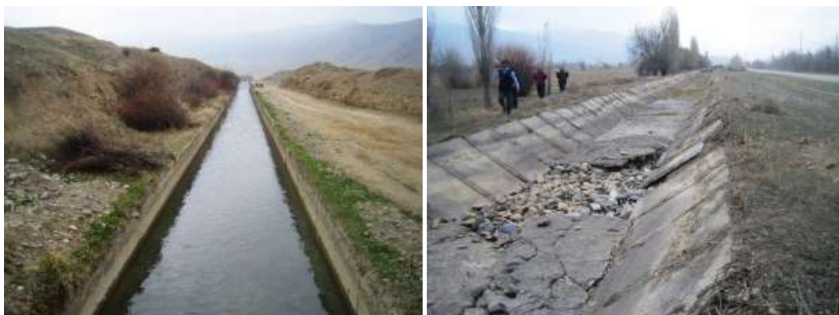
Off-farm canal is very good condition (left) and very poor condition (right)
