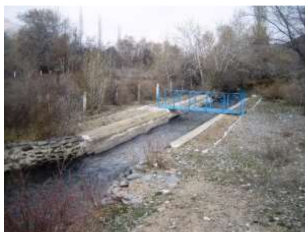
Flow measurement structure at head of off-farm canal
