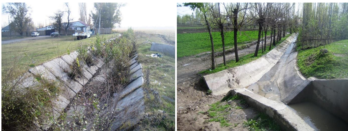
On-farm canal in poor condition in Chui Oblast (left) and in good condition in Jalalabad Oblast (right)
