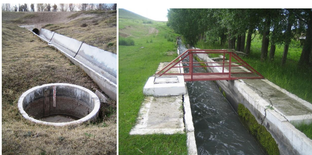
Flow measurement device along on-farm canal in Chui Oblast (left) and Issyk-Kul Oblast (right)
